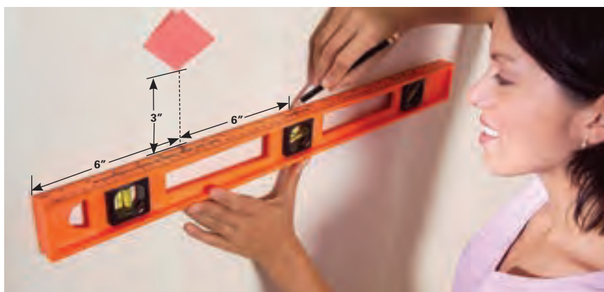
4 Find the hanger positions by measuring down from the sticky note and to each side from center. Keep the hangers level.
